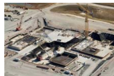
Safety Reviewers Raise Questions about Construction of New Nuclear Fuel Plant
